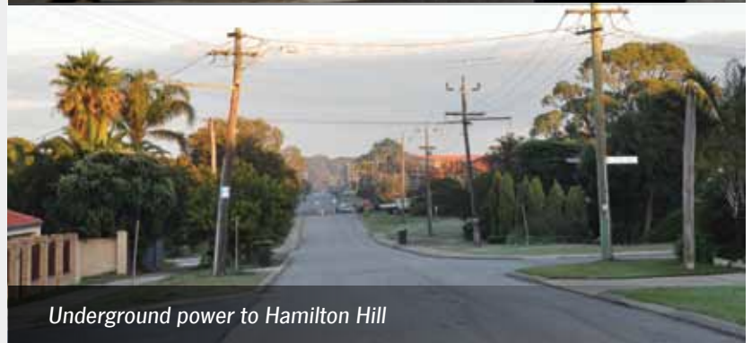
Building roads and infrastructure
