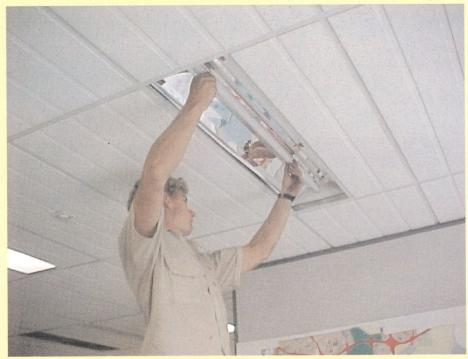
The City of Cockburn undertook a lighting retrofit of the Administration Building in May 2001. This involved removing the existing fluorescent lights and installing a reflective film and electric ballast. This allowed the same light output with the use of only one fluorescent light rather than two. Other measures included replacing existing conventional fluorescent tubes with triphosphorous tubes, which are more energy efficient and have a longer life. The retrofit was an extraordinary success.
